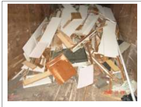
Debris from the demolition of apartment interiors
