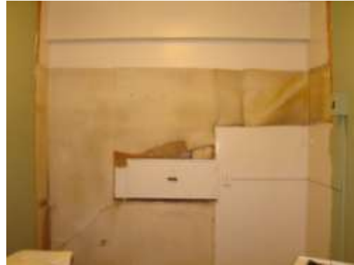
A kitchen after removal of the Hoosier cabinets
